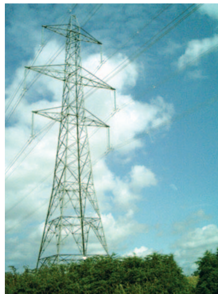
● Fig. 2: A good level of injected power to give a PLT service that works. The distribution of electricity in rural areas is usually achieved on poles and the familiar pylons. Because of this the cables will be natural radiating antenna and the potential for interference to h.f. radio is obvious. Editorial note: The 'Supergrid' system - pictured here in rural Dorset - already radiates r.f. signals (mostly originating from the National Grid's own 'housekeeping' telemetry and switching transmissions) which make themselves known to users of the long and medium wave broadcast bands, particular as you drive under or near them while listening on a car radio! Incidentally, eagle-eyed readers will note that the three phase 'Supergrid' route on the right of this photograph is 'earthed' for maintenance. This pylon - on the section between Mannington Heath Supergrid Substation and Wimborne had many miles of the route out of use and clearly indicated as such by the statutory notices under 'Permit to Work' system for heavy maintenance (each phase is earthed at the individual pylons). The reduction in radiated noise in the l.f., m.f. and h.f. parts of the spectrum were truly dramatic when the photograph was taken on 17 July by G3XFD.
